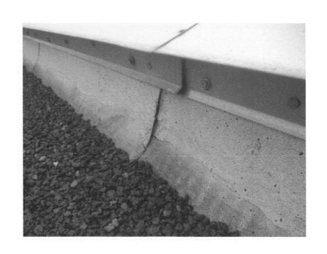
The weather in our region is tough on roofing products. Thermal expansion and contraction as well as UV light exposure cause the roofing plies and asphalt to dry out and weaken. Most roofs in our region are replaced shortly after their 20<sup>th</sup> birthday.
