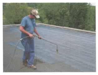
• All loose gravel will be vacuumed from the surface of the roof. An asphalt primer will then be spray applied to promote better adhesion of the restoration material.
