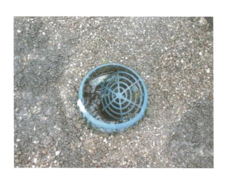
The photo shows the damaging effects of the elements. The plastic roof drain strainer has dry rotted and split. The weather can have the same effect on the waterproofing roofing plies.
