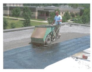
• Once the primer has dried, Garland manufactured "Weatherscreen" is applied at a rate of 8 gallons per 100 square feet. This rubberized asphalt restoration product soaks down into the existing roof to provide additional waterproofing integrity. Slag surfacing is then applied to protect the new roof restoration system.
