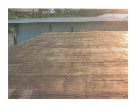
The sun heats up the components of a roof throughout the course of the day. As the sun begins to set, roof surface temperatures will cool fairly evenly with the exception of any areas that contain moisture. The wet roof insulation boards retain the heat of the day longer and can be identified with the thermal imaging equipment.
