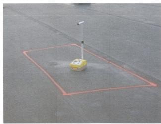
All areas of wet roof insulation will be marked on the roof in architectural paint.
